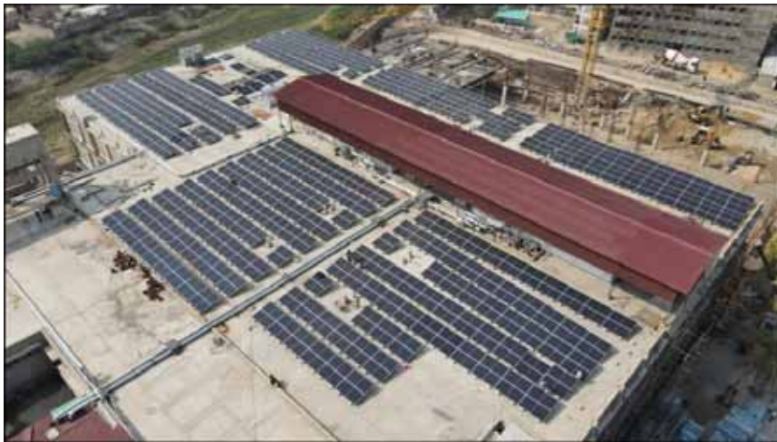
Solar plant installation at Gatron (Industries) Limited
